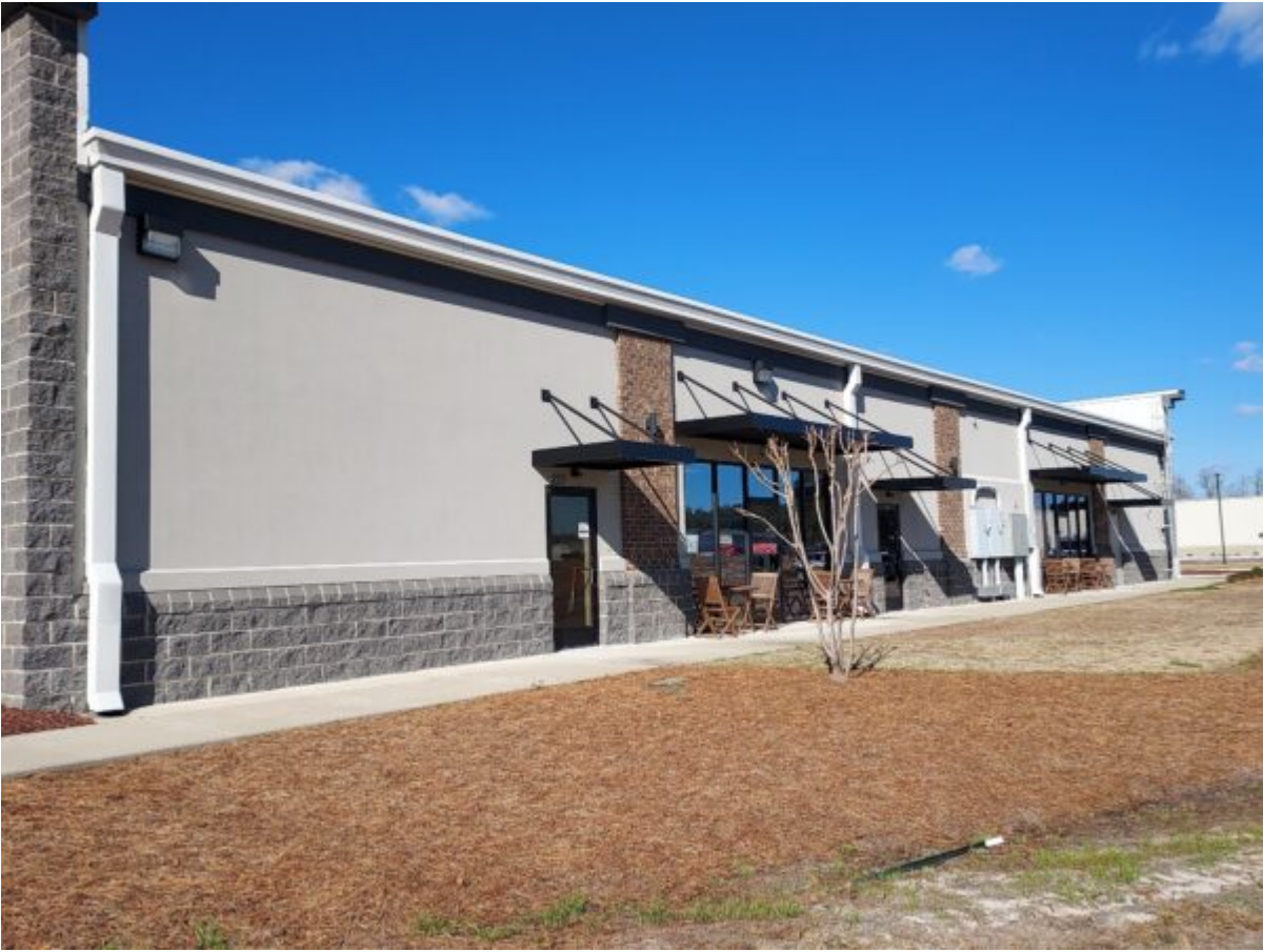
Front View of Building View
